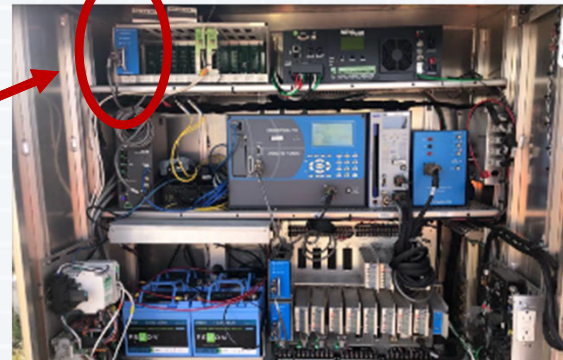
Signal Command Module Communicates with signal controller and fiber
