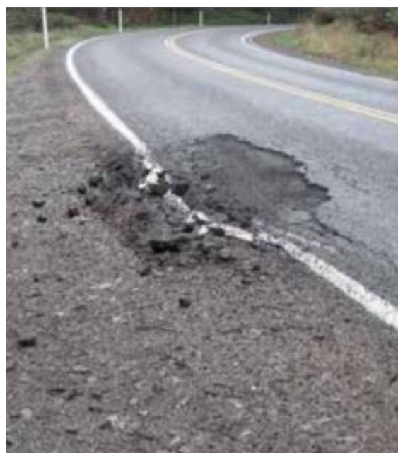
Figure 2-5: Pavement Damage at a Truck Pull Out
